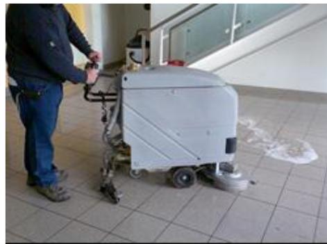
c) Finally swill the surface with clean water to remove the residue and then dry the floor by squeegee or wet vacuum. The surface should then be allowed to fully dry.
