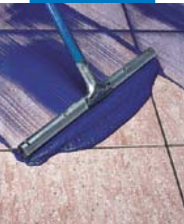
Grouting a porcelain tile floor with a float
