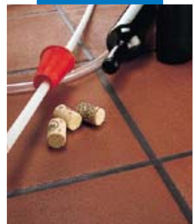
An example of a grouted terracotta wine-cellar
