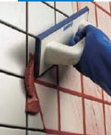
Grouting a wall with a rubber float (bathroom or kitchen)
